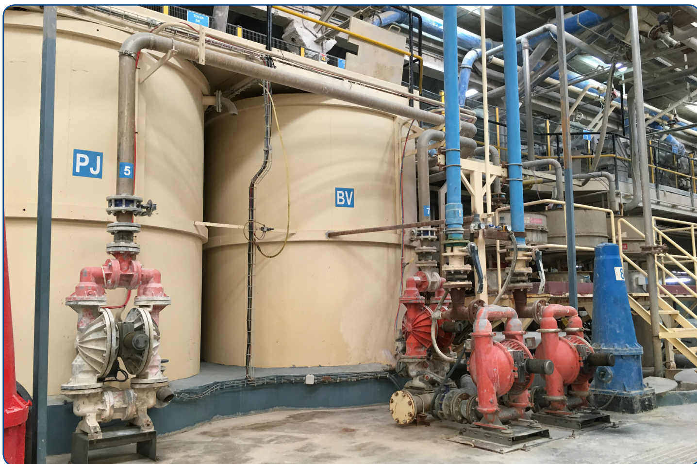
Wilden® Original™ Series Air-Operated Double-Diaphragm (AODD) Pumps in operation at a ceramic plant in Spain.
