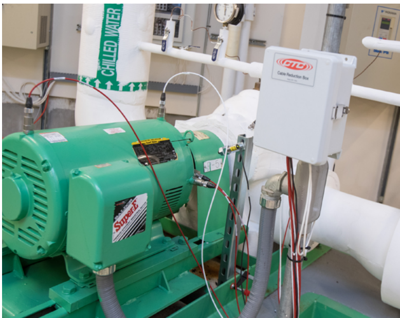
Equipment monitoring systems are used to detect trends and anomalies for accurate diagnosis.
