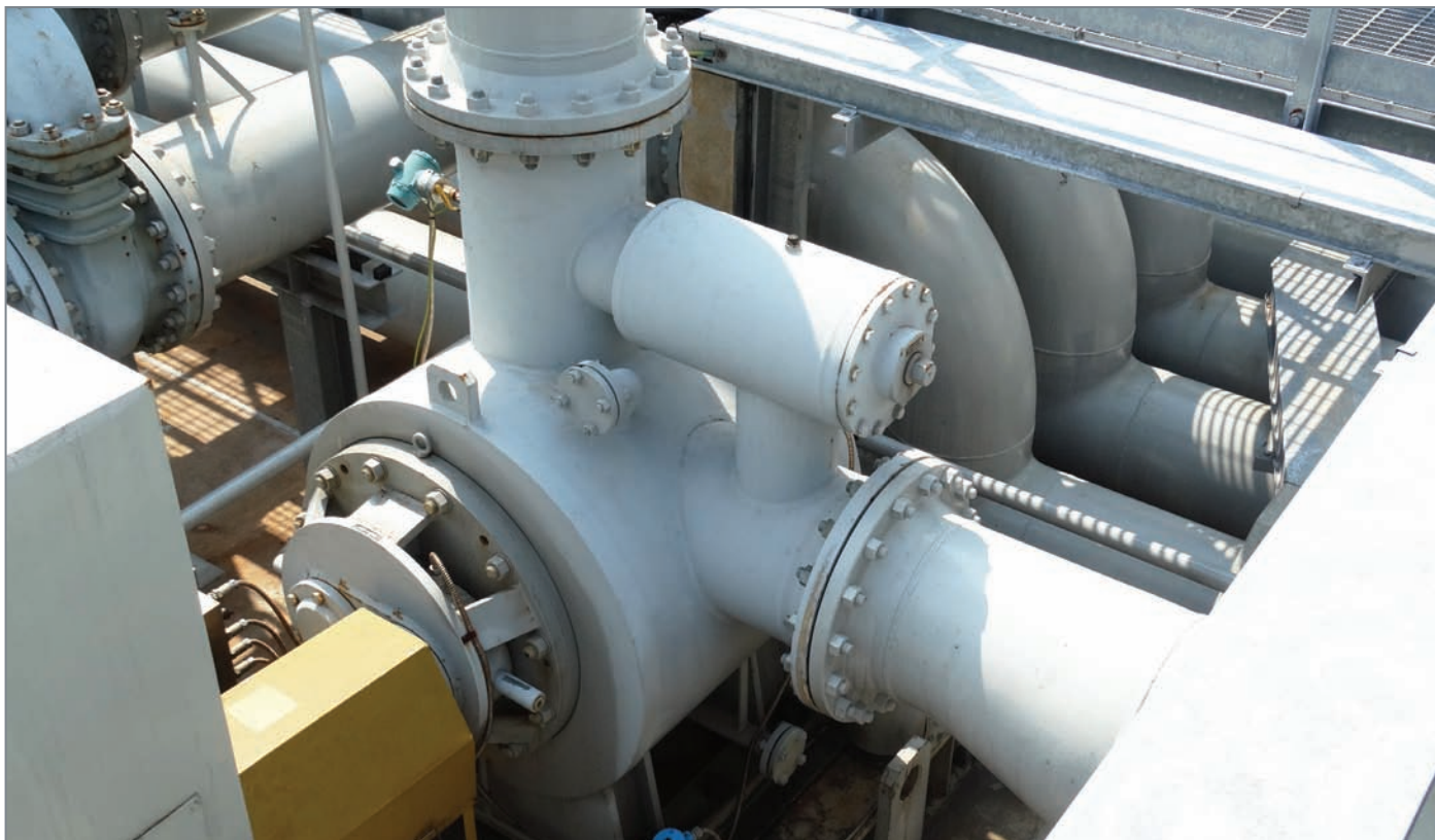
Rotary positive displacement (PD) pumps installed in a process pumping system. Shown are Blackmer® S Series screw pumps.
